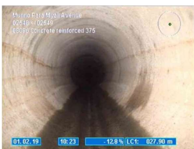
Pipe in good condition
